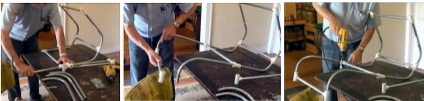
4. Next, insert the four medium bends (long end toward the "U"). On one side, point the two curved parts of the medium bends downward and add a tee-post to keep alignment correct. Insert a screw on each of the tee posts where the long end is connected. Do the same thing on the other side. Now put a screw into the tee posts adjoining the curved part of the medium bends. See illustration.
